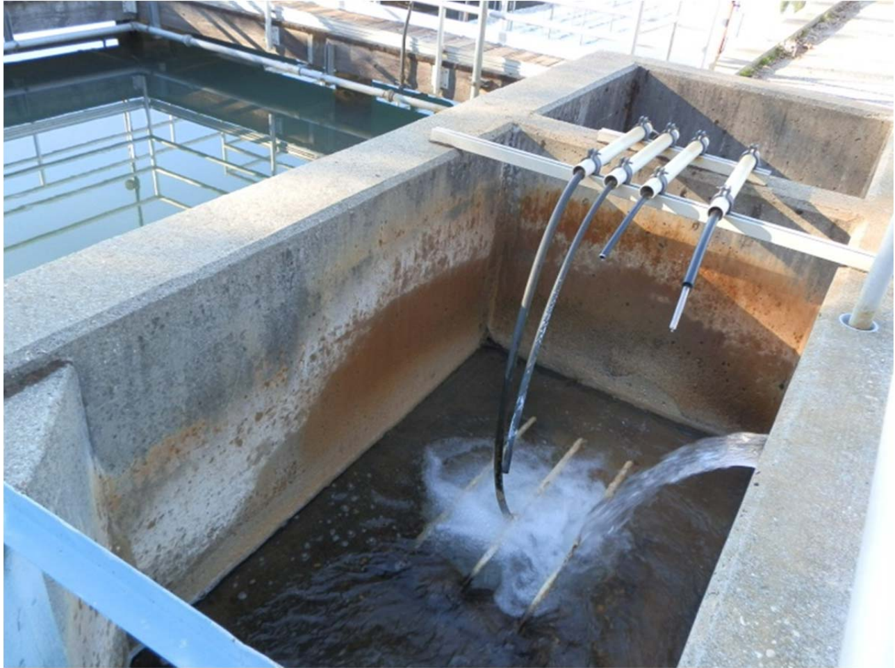
Figure 5-4 Chemical Injection
