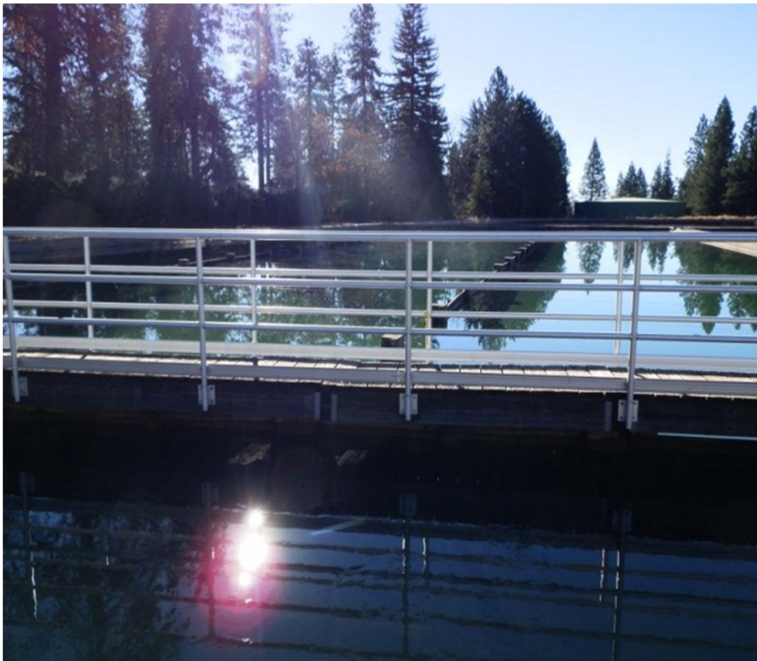
Figure 5-14 Existing Catwalks between the Sedimentation and Flocculation Basins
