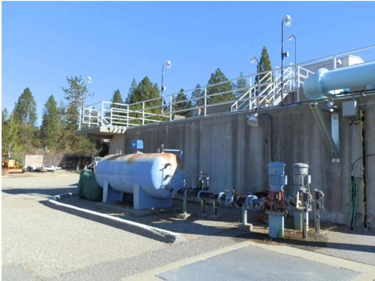
Figure 5-13 Plant Water System
