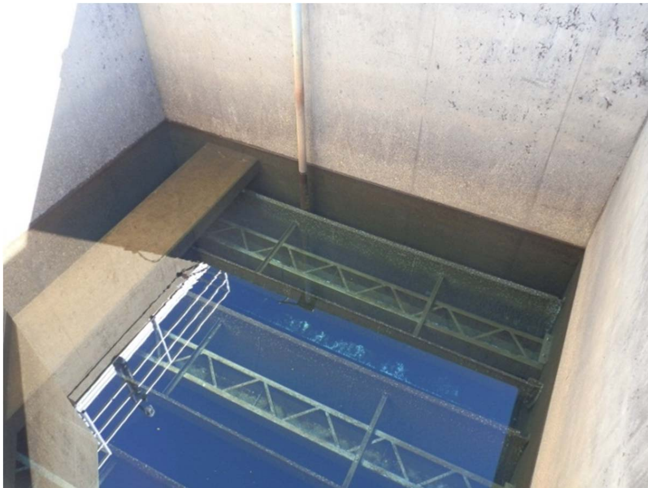
Figure 5-8 Filter Basins
