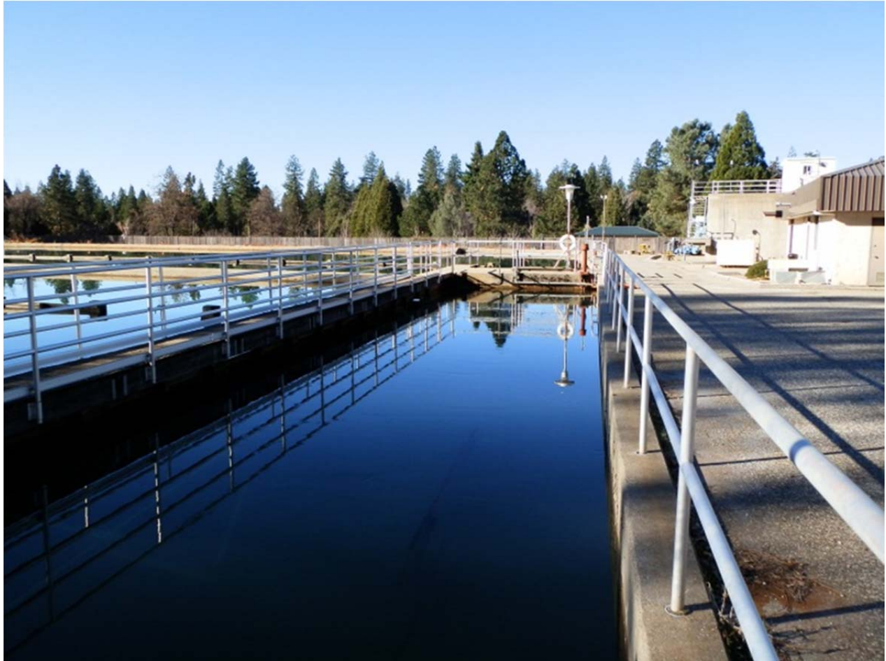
Figure 5-5 Flocculation Basin
