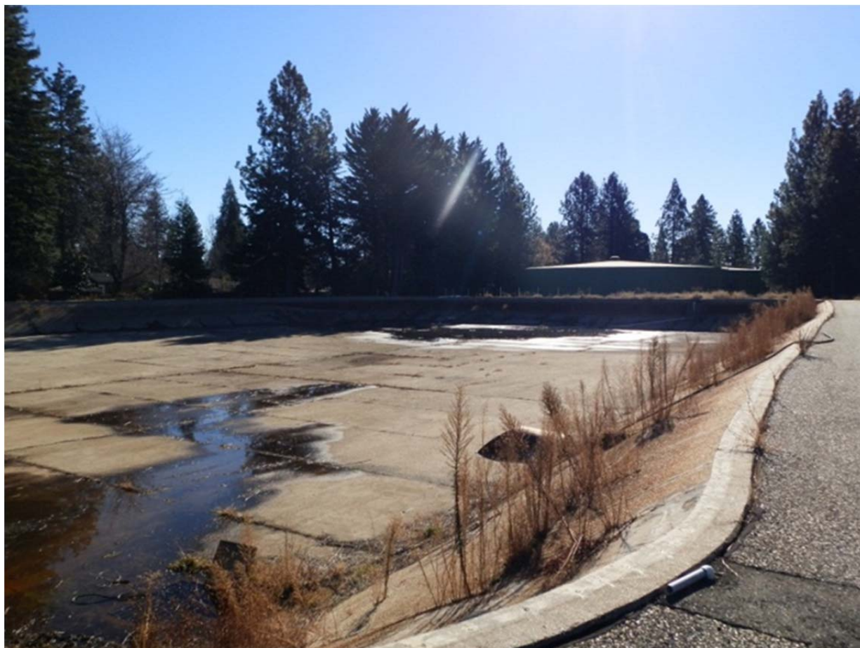
Figure 5-12 Old Treated Water Reservoir (Old Storage Basin)
