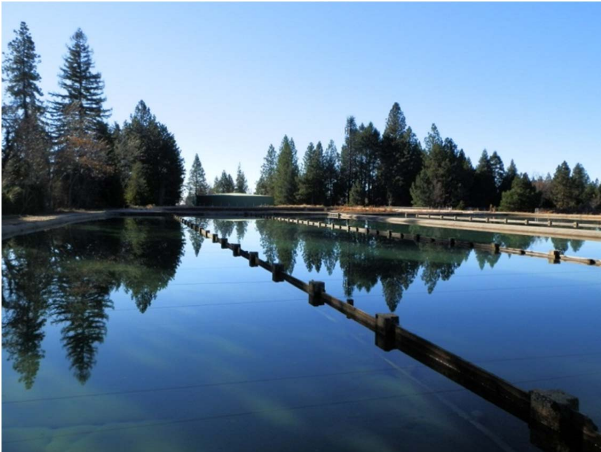
Figure 5-6 Sedimentation Basin
