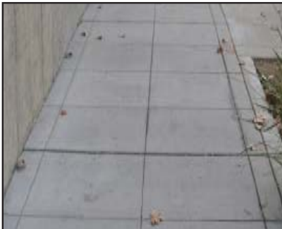
Concrete Paving 2' x 2' score pattern
